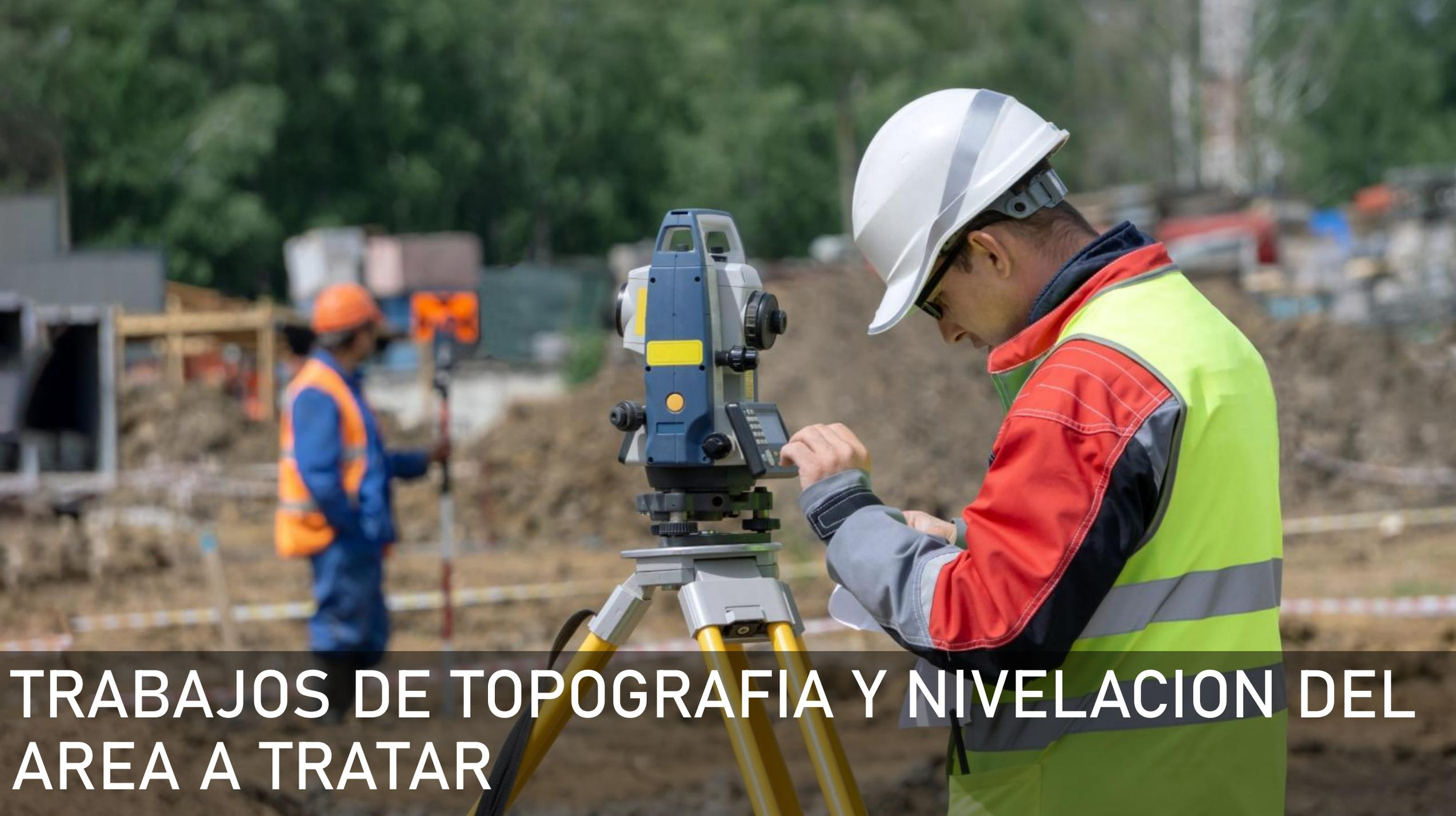
A surveyor wearing a white hard hat and a high-visibility vest is operating a total station on a tripod. The background shows a construction site with another worker in the distance.
