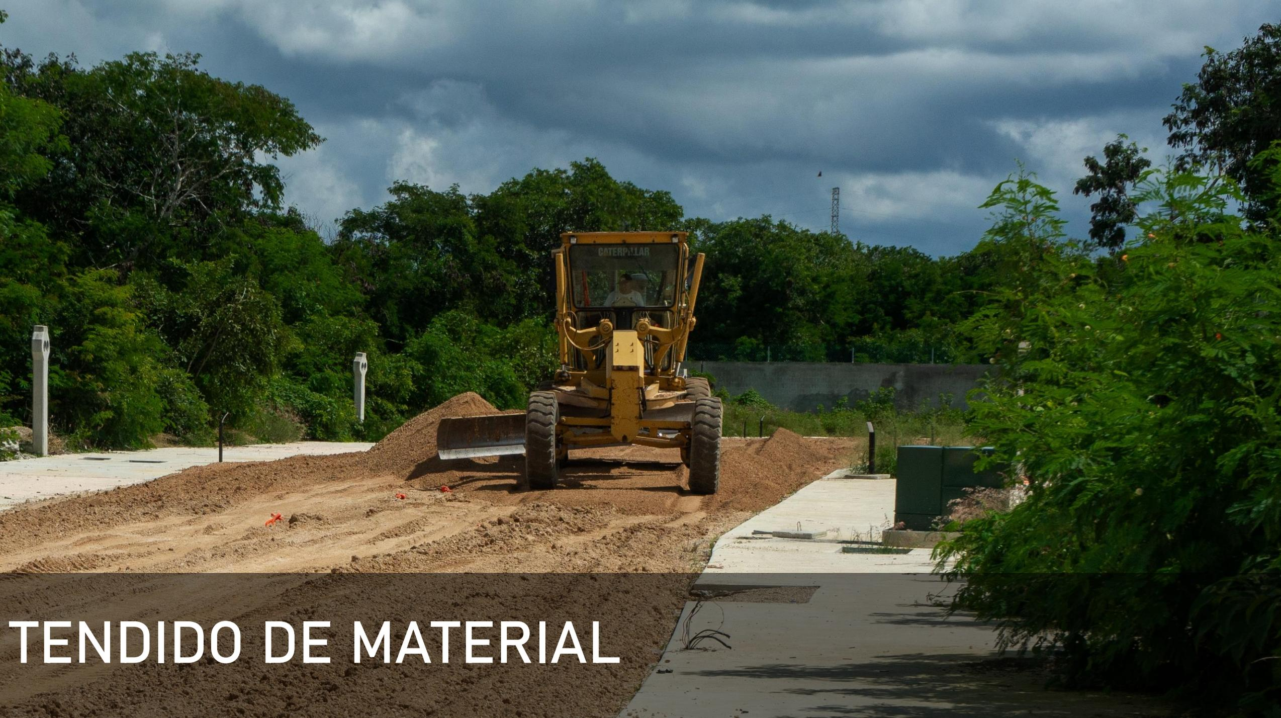
A yellow Caterpillar motor grader is shown from a rear perspective, spreading a layer of brown material (likely soil or gravel) onto a prepared surface. The machine is positioned on a dirt path that runs alongside a concrete curb. In the background, there is a dense line of green trees and a cloudy sky. A utility tower is visible in the distance. The scene is set in a construction or landscaping area.
